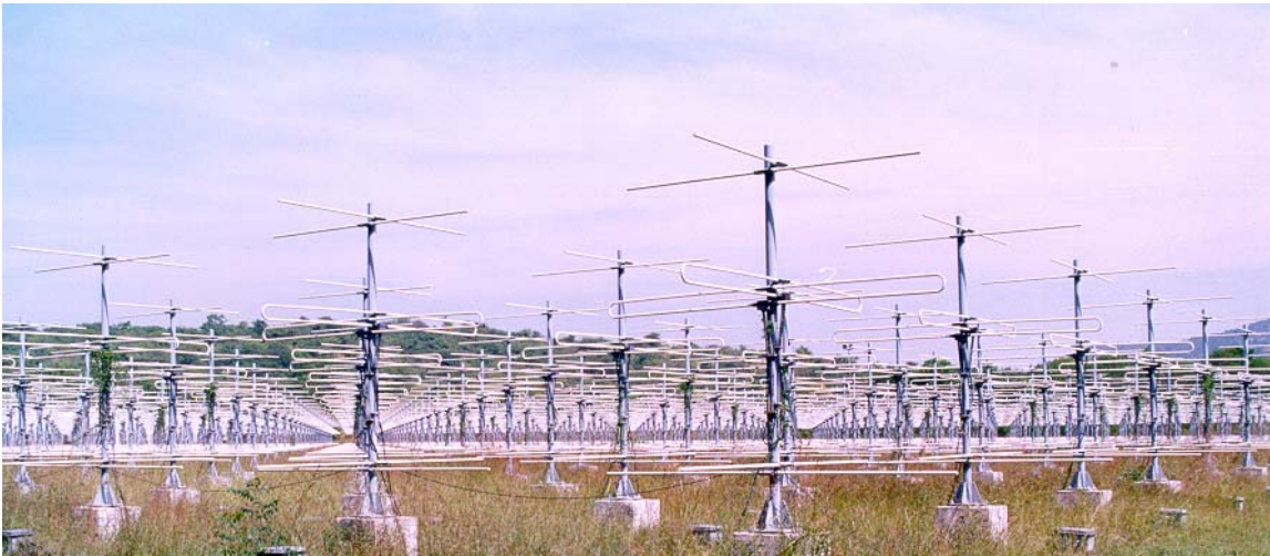
Figure 2.7: View of the individual three-element crossed Yagis from antenna array floor.
