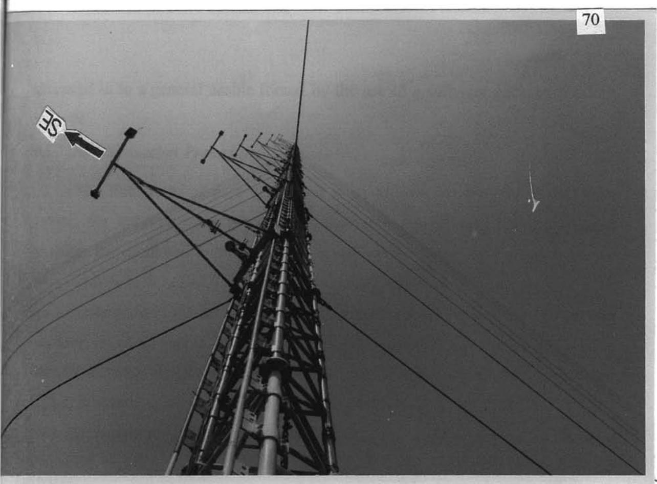
Figure 3.4 100 m tower structure showing insrument arms and guy wires
