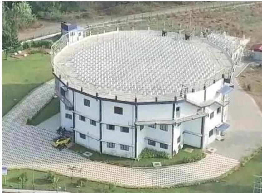
Fig. 2.3: ST radar Facility at ACARR
